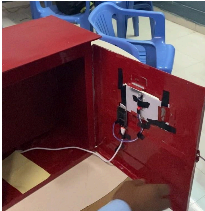
Figure 2. View of Inside
